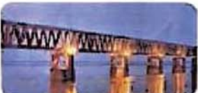
More than 80% of SAIL steel used in Boghead Bridge, Assam. It would be longest rail-rum road bridge in India.
