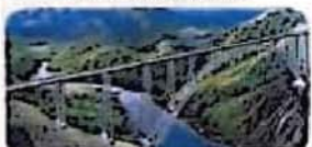
SAIL supplied materials to Chenab bridge (The World's Highest Rail Bridge constructed in India)
