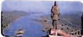
12000 metric tonnes of SAIL steel (more than 36 percent) used in construction of 182 meters tall 'The Statue of Unity', The World's Tallest Statue
